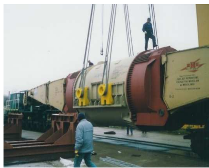
Fig.4. Unloading 330 ton generator from wagon type NORCA
