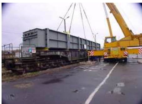
Fig.3. Transportation of machine unit for refinery
